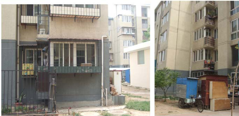
Figure 5. The drainpipes installed from the second or third floor
