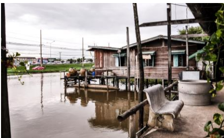
Waterside image before flood barrier.
