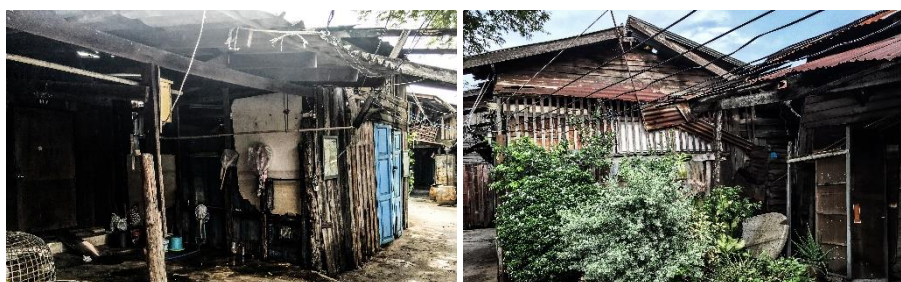
Decadence due to living activities
