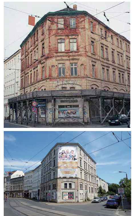
图3 莱比锡戈利斯村街角建筑改造前后对比图 Fig.3 comparison of the corner building before and after the renovation in Gohlis village, Leipzig
