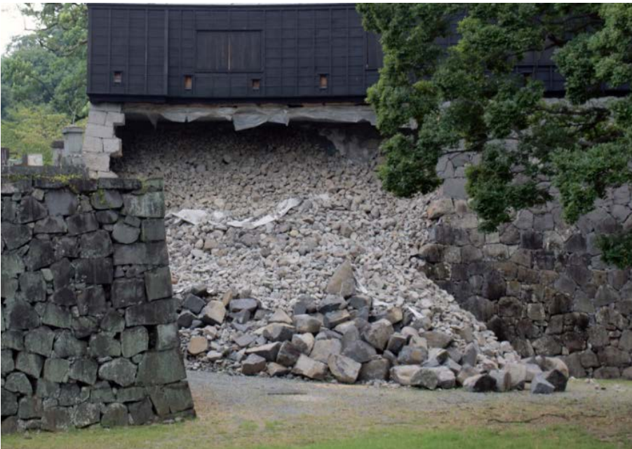
Figure 2. A Collapsed Wall at Kumamoto Castle (Photo by Kimihide Yamamoto on Aug. 2016)
