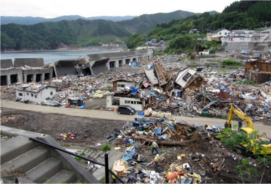
Figure 1. Damage to A Large Embankment (Photo by Ryohei Yamashita on June 2011)
