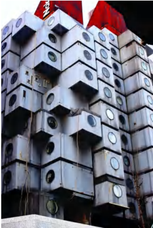
• Prefabricated container residence
