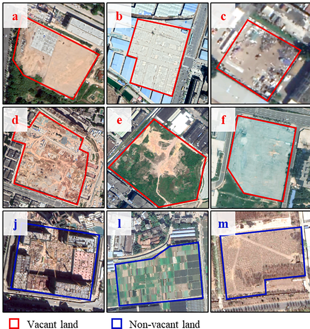
Fig. 3. Examples of vacant land and non-vacant land with similar features. (a) is bare land without film and weeds. (b) is land with demolished structures. (c) is the derelict hardened ground with garbage. (d) is land under early-stage construction. (e) is land with weeds. (f) is bare land covered with green film. (j) is land under late-stage construction. (l) is green farmland. (m) is brown woodland.
