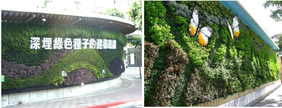
Figure 2. Example of vertical greening on construction fences in Taipei
