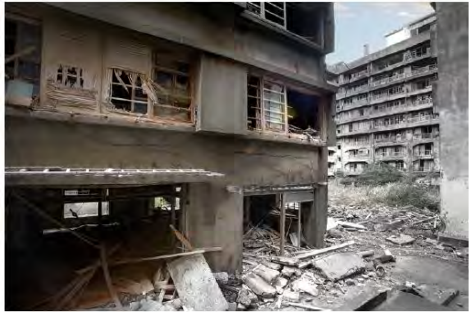
Fig. 7.1 Ruined housing on Hashima Island (Photo by Ott Kadarik)
